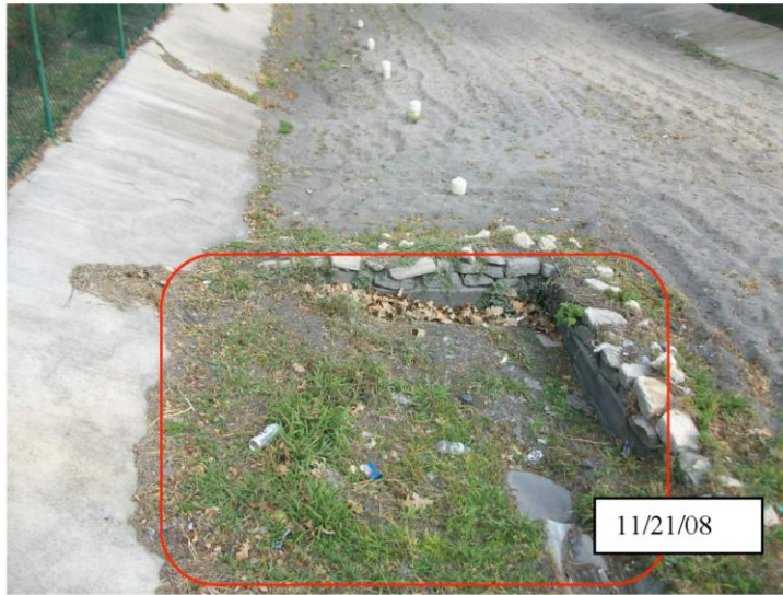
While inspecting the basin the inspector found heavy accumulation of sediment, debris, and vegetation within the splash pad.
