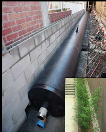
cisterns at NRDC santa monica office
