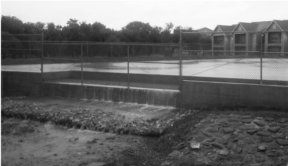
Figure A.2.3: Structural BMP (sand filter) near the South Boundary of the UTSA main campus Source: With Permission from the UTSA Office of Facilities (2015)
