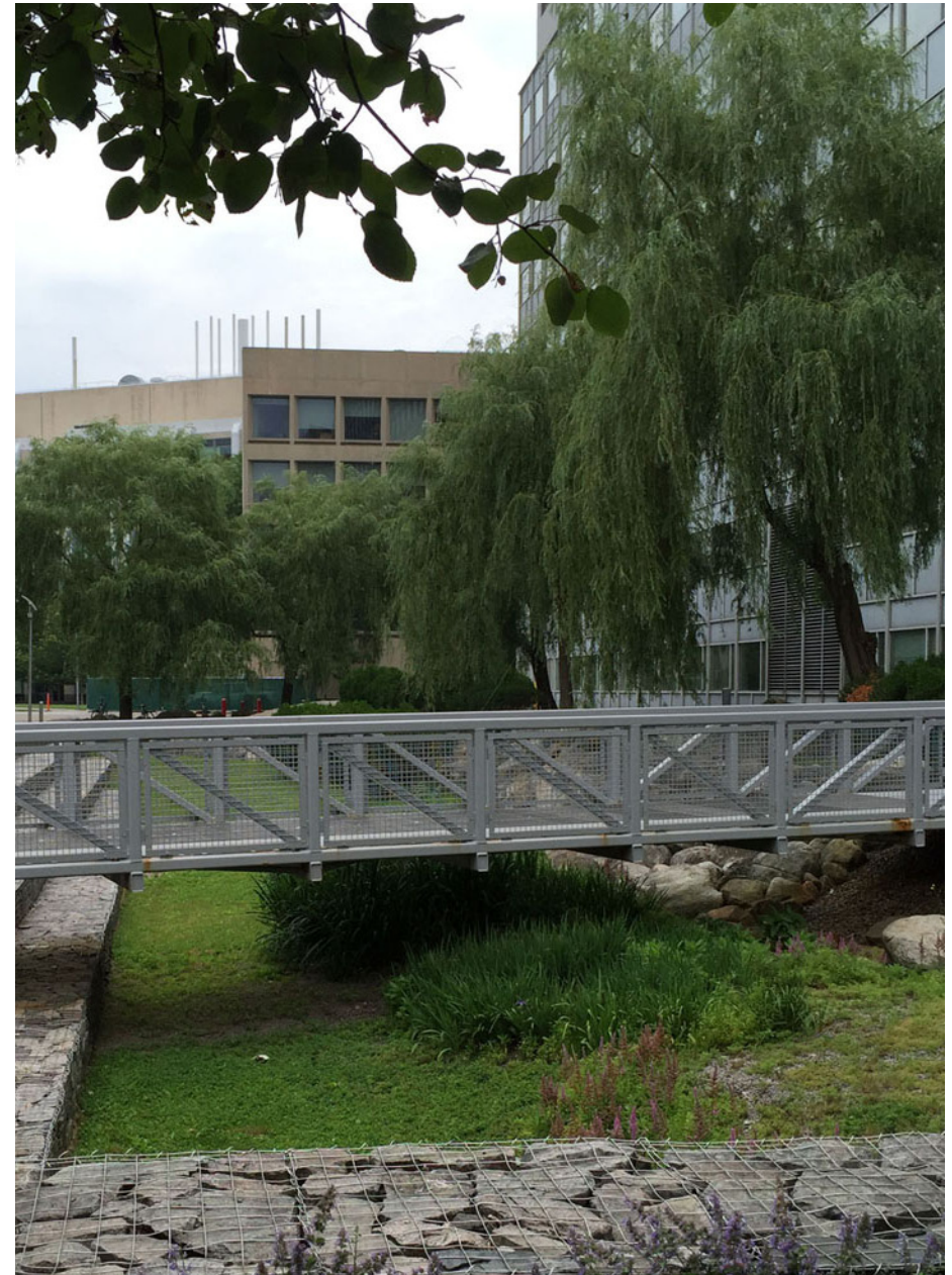
Figure B.3.2: Vegetated Swale in the MIT Campus, Cambridge, Massachusetts.
