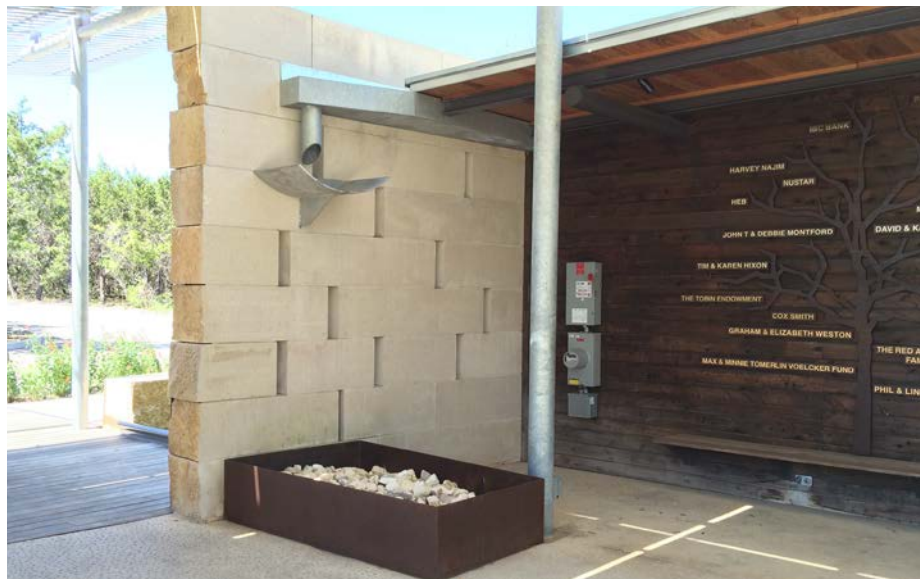
Figure B.2.14: Rainwater Harvesting, A Container Directs the Water to Underground Cistern, Phil Hardberger Park, San Antonio, Texas.
