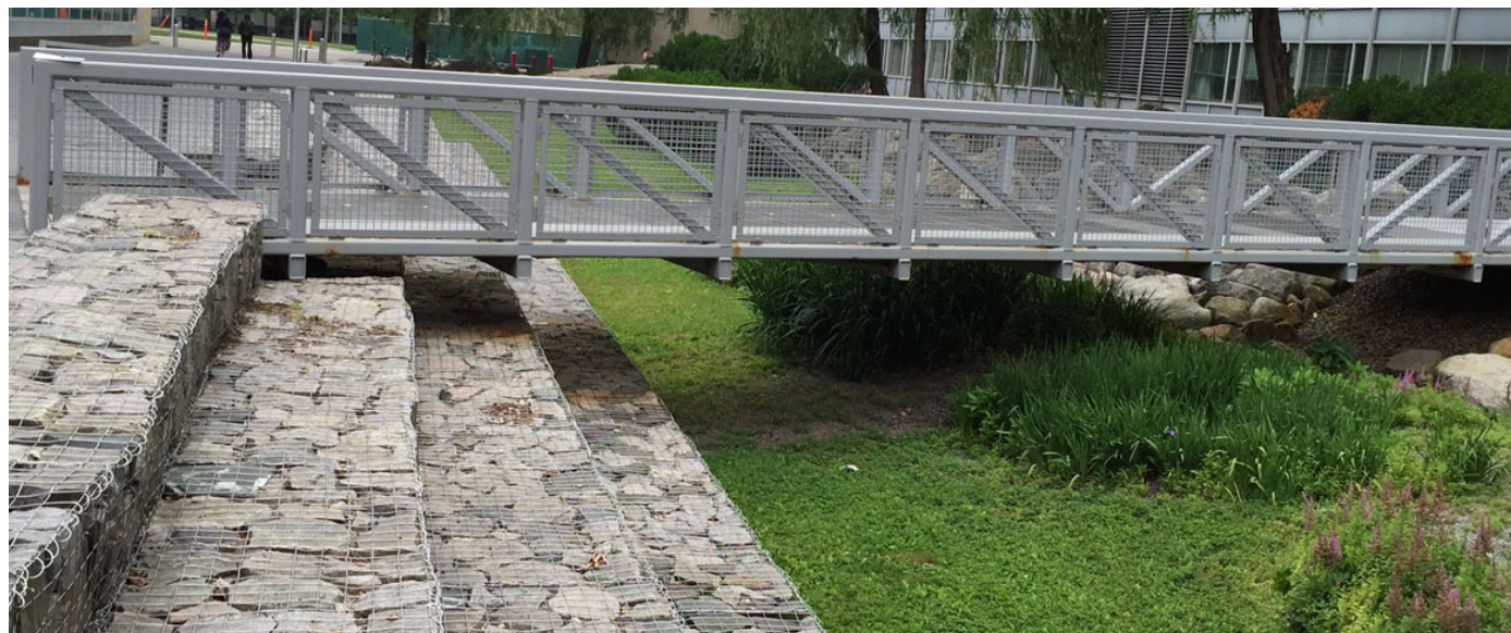
Figure B.2.8: Vegetated Swale in the MIT Campus, Cambridge, Massachusetts.
