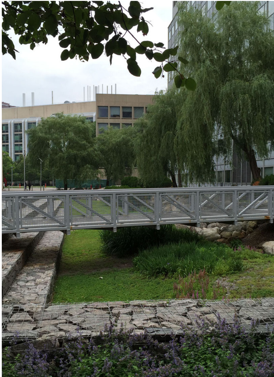
Figure B.2.1: Vegetated Swale in the MIT Campus, Cambridge, Massachusetts.
