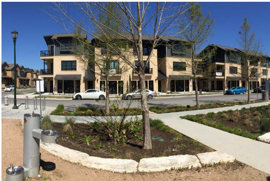
Figure A.3.2: Rain Garden at Mueller Community, Austin, Texas.
