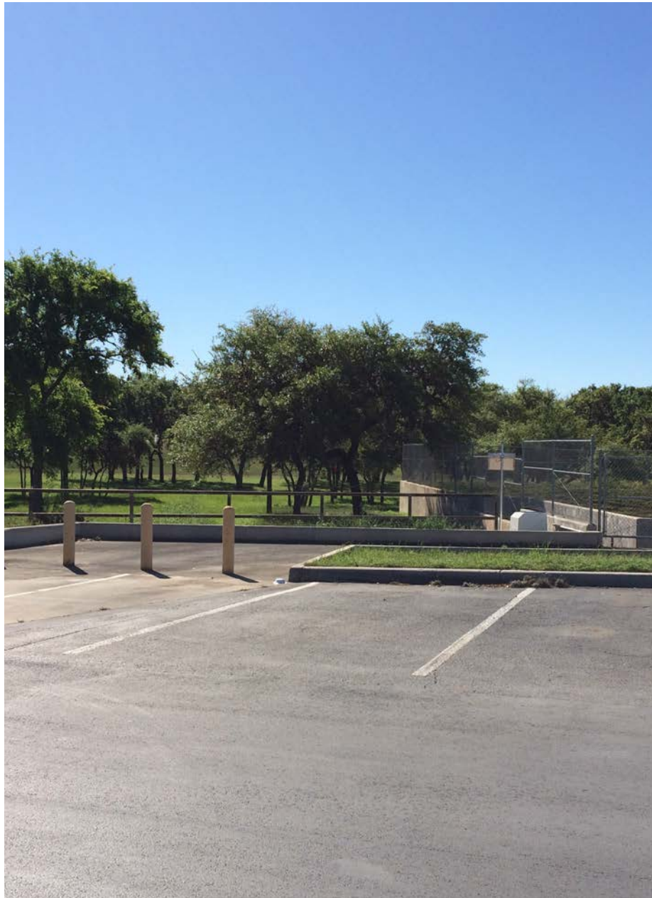
Figure B.3.10: A structural BMP (sand filter) located in the south boundary of the UTSA main campus in San Antonio, TX
