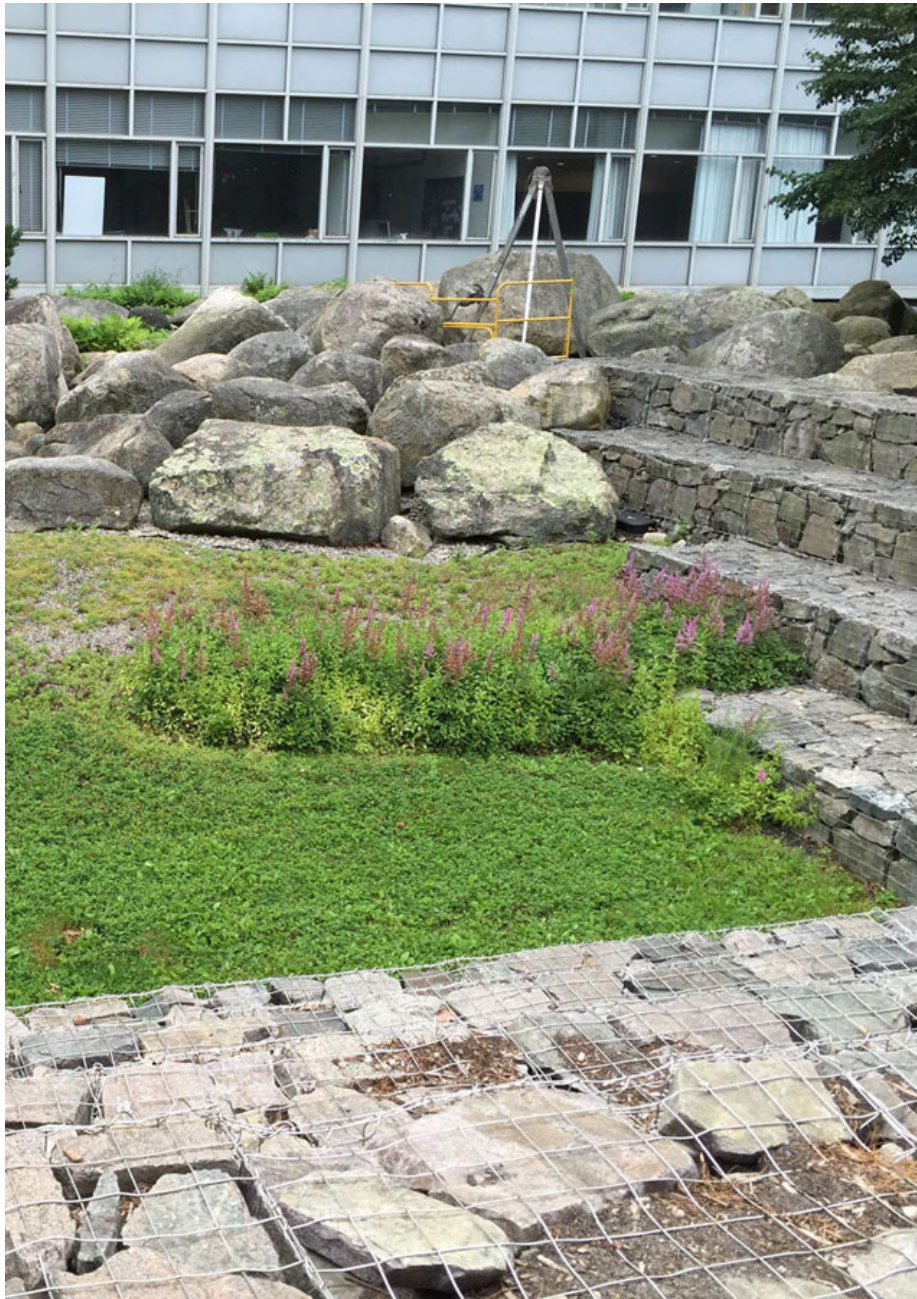
Figure A.5.1: Vegetated Swale in the MIT Campus, Cambridge, Massachusetts.
