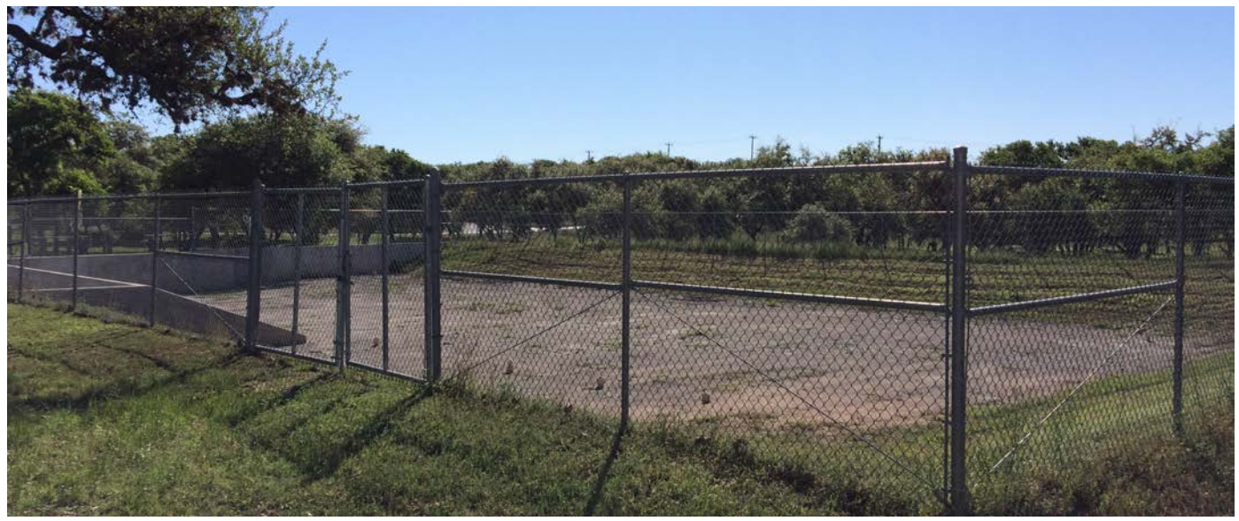
Figure B.2.9: Sand Filter in the main campus at UTSA, San Antonio, Texas.
