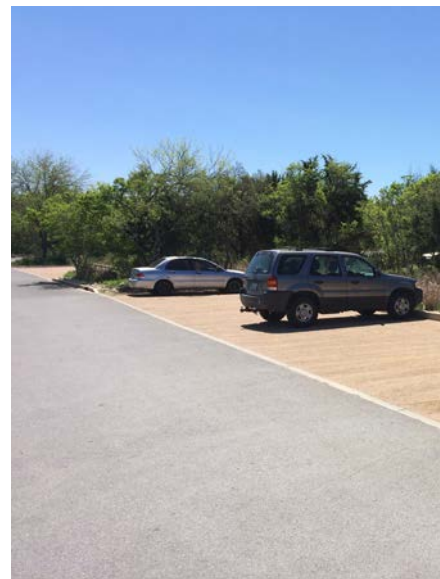
Figure B.2.11: Permeable Pavement in Phil Hardberger Park, San Antonio, Texas.
