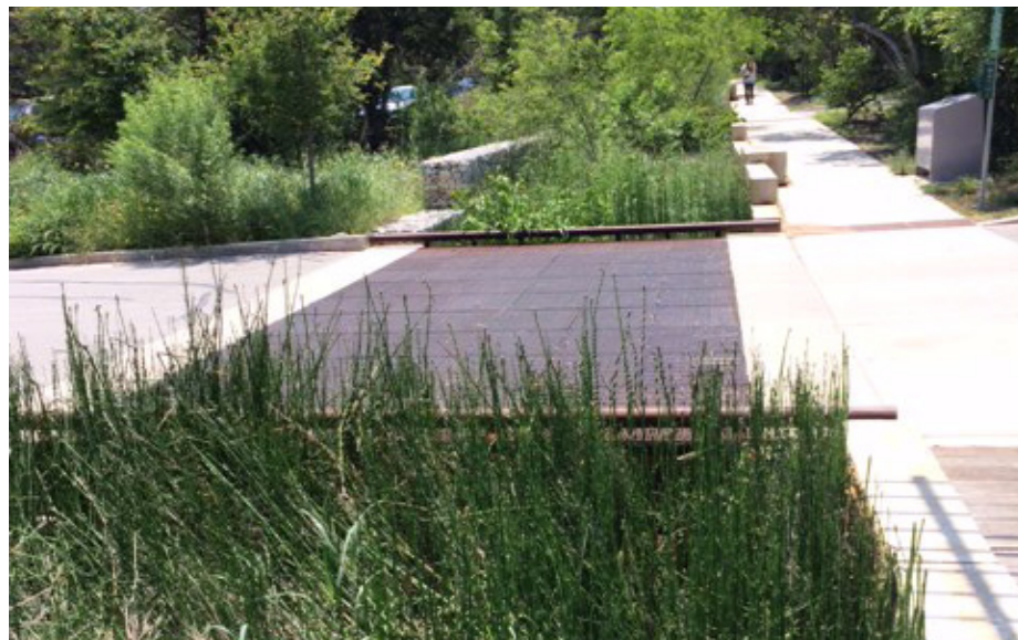
Figure B.2.6: Bioretention Swale located in Phil Hardberger Park, San Antonio, Texas. Source: with permission of San Antonio River Authority SARA (2016)
