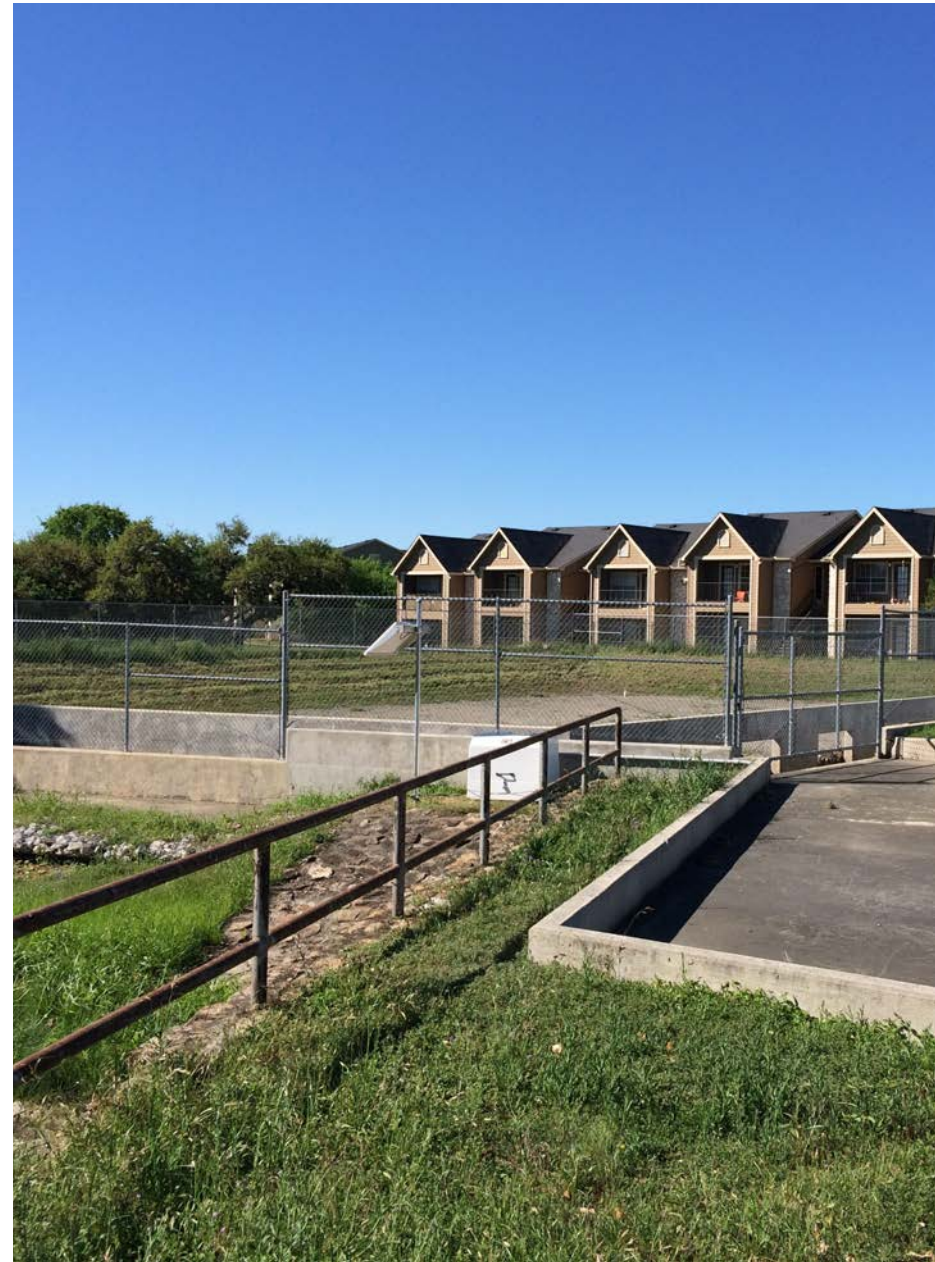
Figure B.3.1: A structural BMP (sand filter) located along the southern boundary of the UTSA main campus in San Antonio, TX
