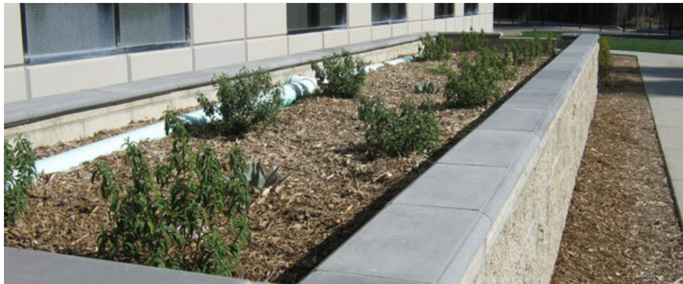
Figure B.2.13: Above ground flow-through planter at the Riverside County Flood Control and Water Conservation District, Riverside, CA Source: http://countyofriverside.maps.arcgis.com/apps/MapTour/index.html?appid=23596d603ef14c128e765ac698e54f8c#
