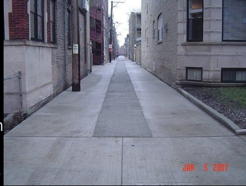
high albedo concrete and permeable concrete trench in chicago alley. photo courtesy of abby hall, u.s. epa.
