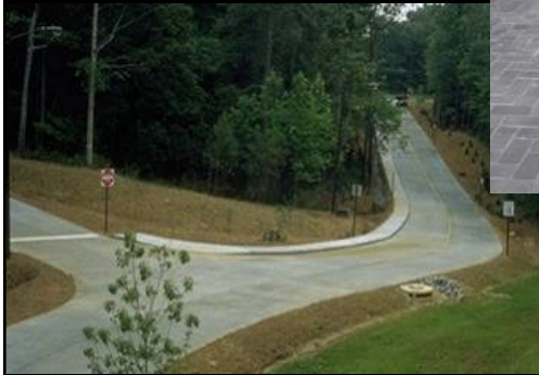
permeable concrete – webb bridge park, alpharetta, georgia.
