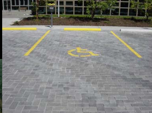
ada compliant interlocking concrete paver blocks. portland, oregon.
