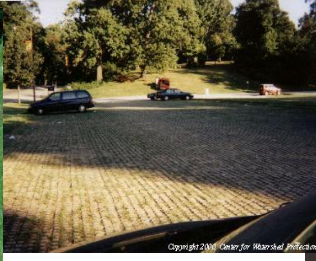
Pervious parking lot
