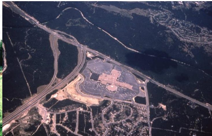
Sand filter – Barton Creek Mall
