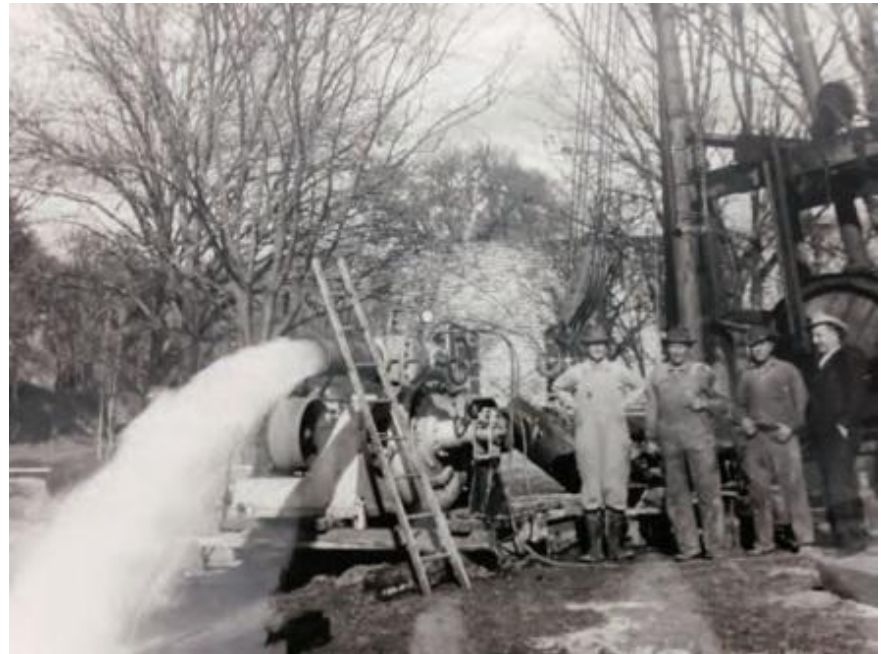
Drilling the third well, December 1944. The water pressurization building is visible in the background.
