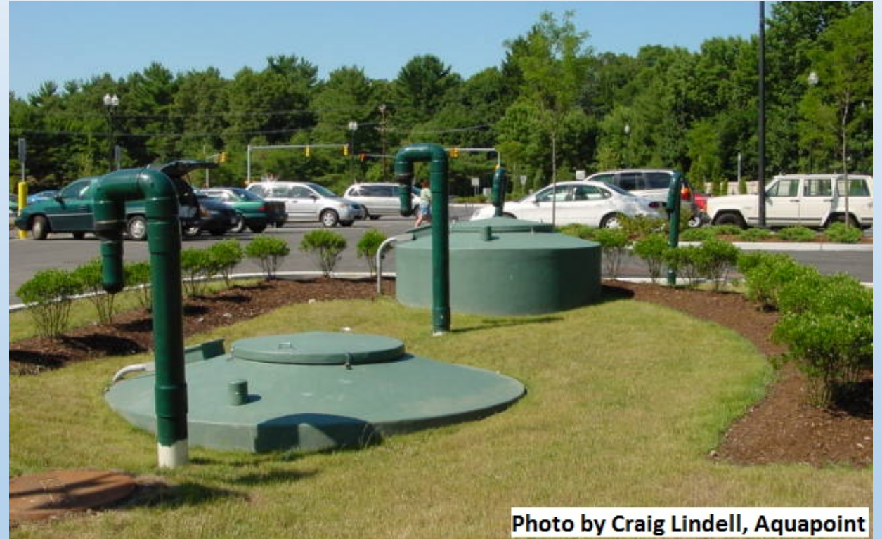
Fixed Film / Attached Growth (Recirculating Trickling Filter) Category of Treatment
