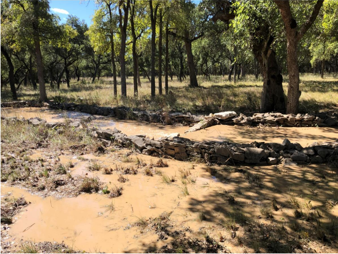
Figure 3 October 25, 2019 photograph of storm water flowing across Langford Property, downstream of property line.
