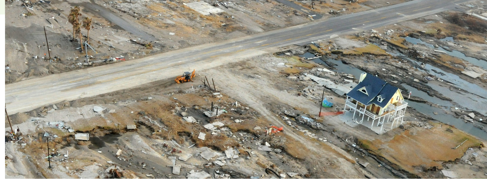
Damage from Hurricane Ike in Texas in 2008. Photo: Federal Emergency Management Agency
