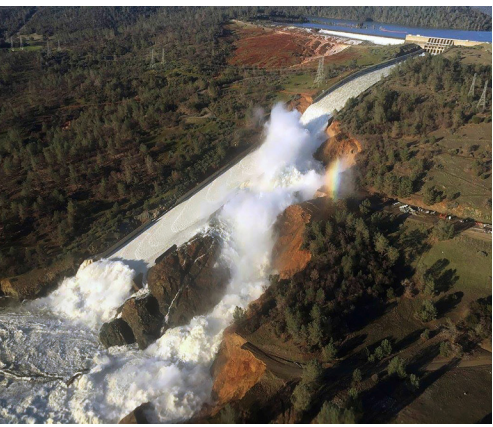
2017 Oroville Dam spillway failure in California. Photo: William Croyle/California Department of Water Resources
