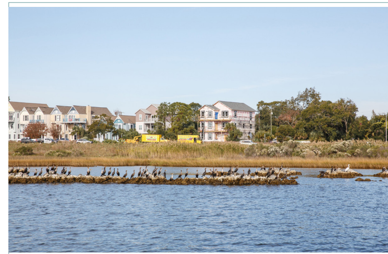
A living shoreline with an offshore oyster reef in Florida attracts wildlife and protects the shoreline. Photo: Kaila Drayton, NWF.
