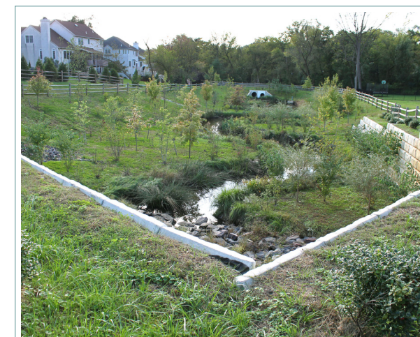
Andorra Creek floodplain restoration. Photo: Montgomery County Planning Commission
