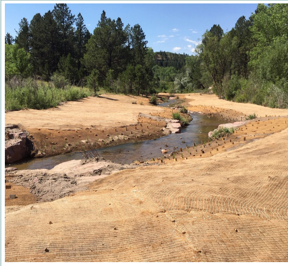
Kettle Creek restoration, Colorado Springs, Colorado. Photo: U.S. Fish and Wildlife Service
