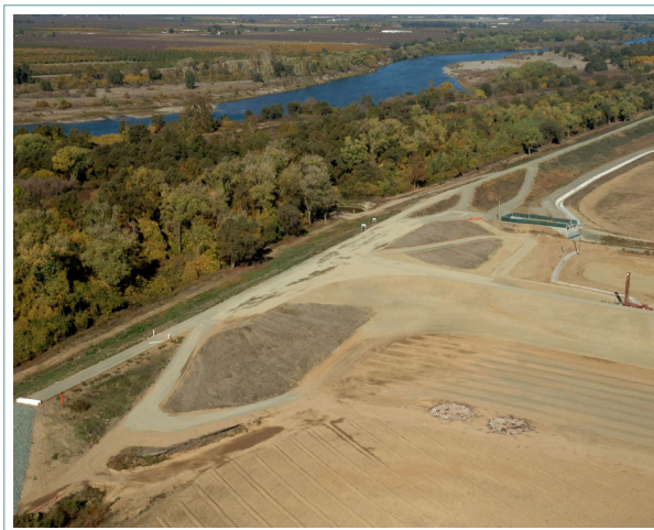
Bear River setback levee in California. Photo: California Department of Water Resources
