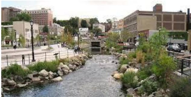
Daylighting a stream
