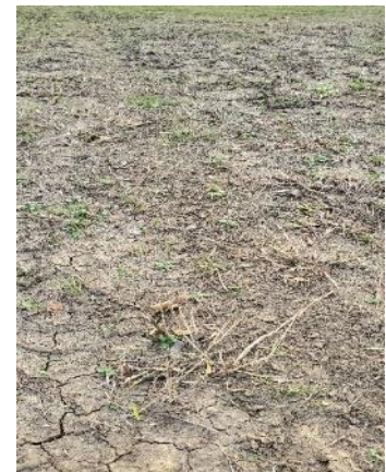
Figure 14: Soil surface crust created by mowing regime, erosion and drought.
