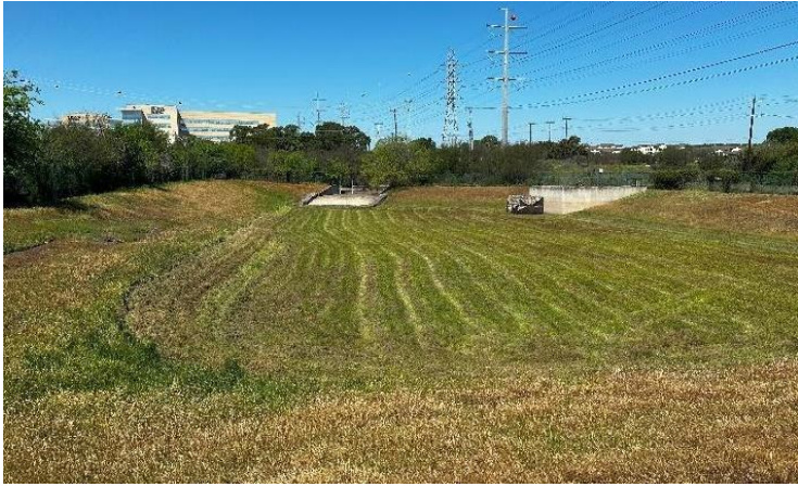
Figure 18: Sand filtration system properly maintained; no standing water, tree seedlings or debris. The turf height is also good.
