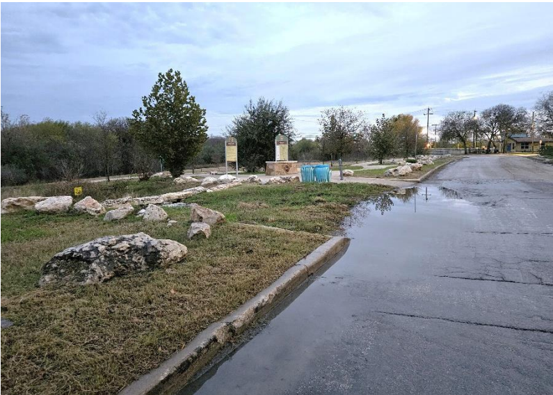
Figure 17: Silt removal is required to allow stormwater to enter the turf area.
