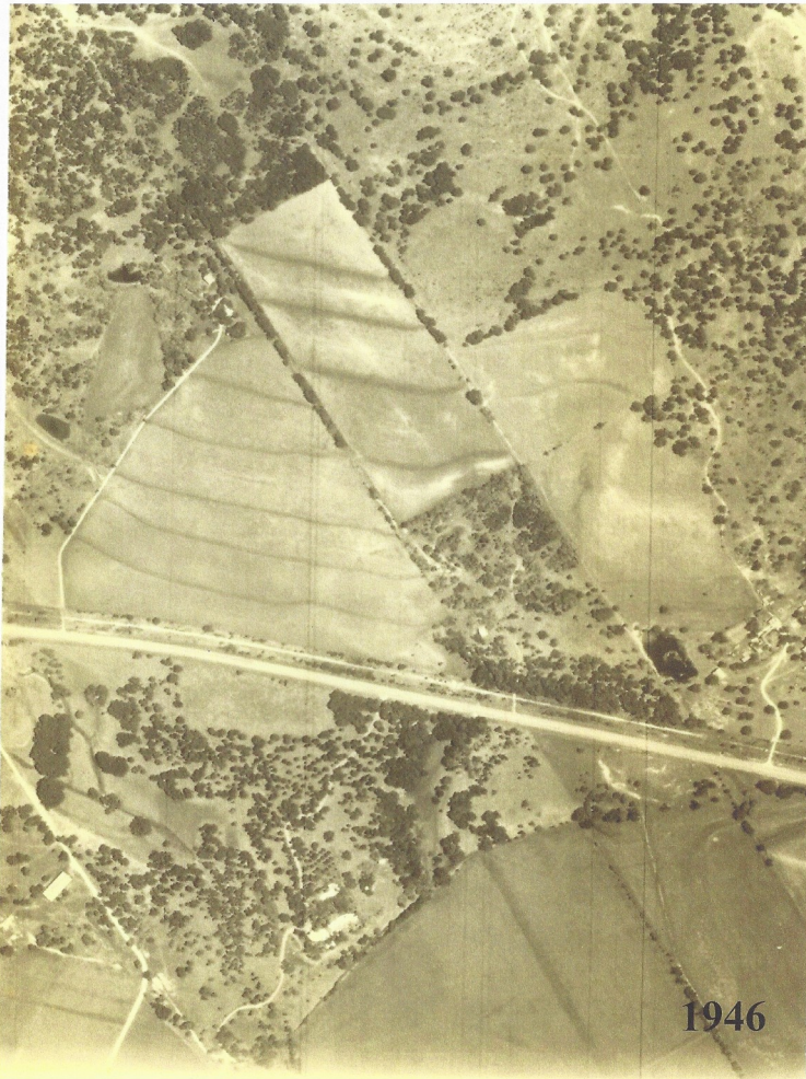
Very fine aerial photograph of the area, with high resolution, taken during the construction of the H.M. Naylor Ranch house c. 1946. The construction of the airport was begun in 1942, but it is still to the west, and not visible in this photograph. Same view is shown on the right, with "craters" delineated. Photo: Naylor Ranch Archives.
