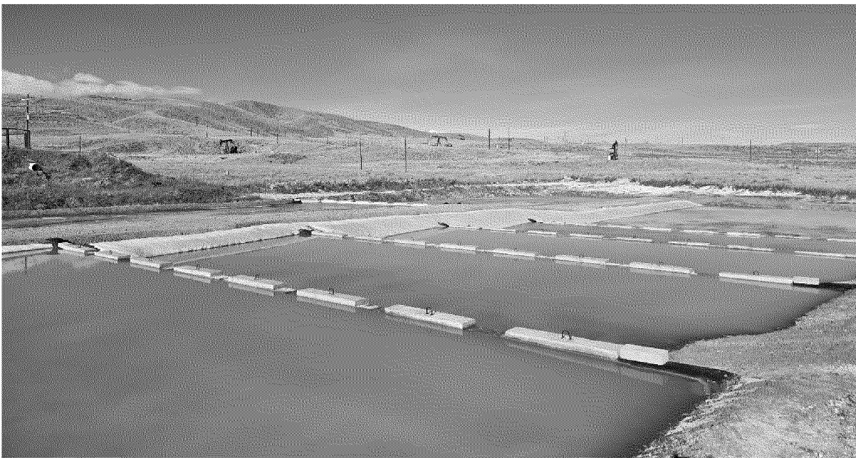
Figure 6. Sulfides Treatment Basin at a Wyoming Production Site
