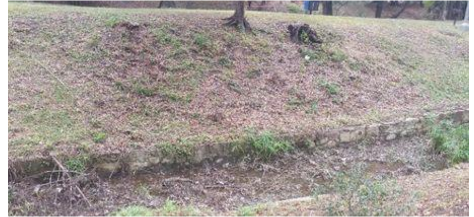
Vegetation cut too short increasing soil erosion and weeds.
